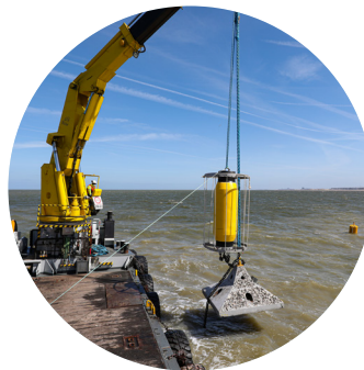
Single mooring mussel shaker during installation.
