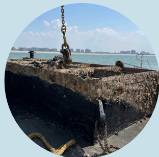
1 out of 6 backbones were anchored by means of 2 different gravity anchors of approximately 15-16T.
