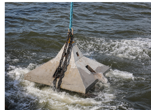
Bio-facilitating anchor during installation.
